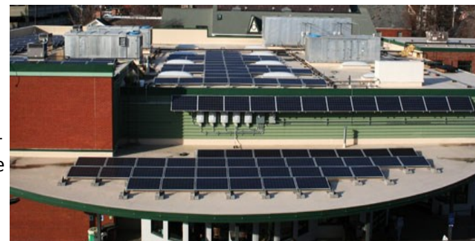
City Market Solar Panels
