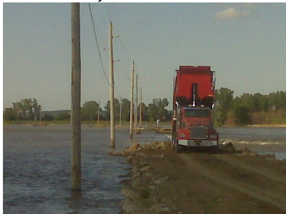
Figure 3.24. Missouri River Flooding 2011 – Leavenworth County
